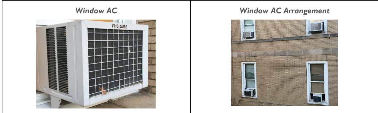
Figure 10 – DX Air Conditioning System
